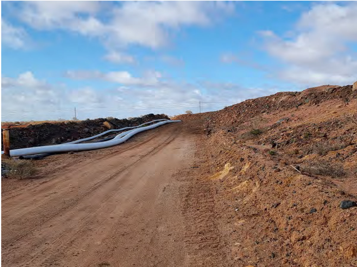
Photo 7. Road of South Pit - looking South-East
