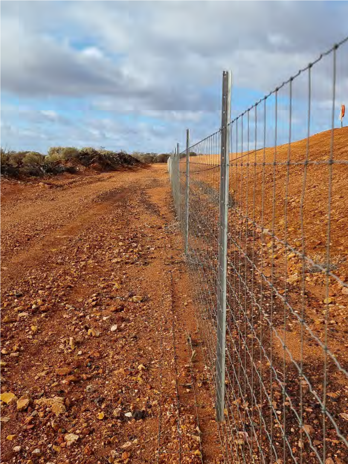
Photo 2. WMP8 (Area 2) – looking South East
