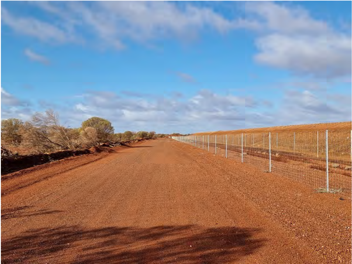
Photo 4. WMP9 (Area 1)- looking South-South-East
