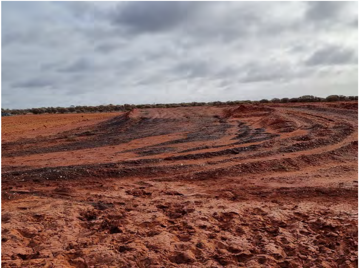
Photo 1. Topsoil (Area 3) – looking North
