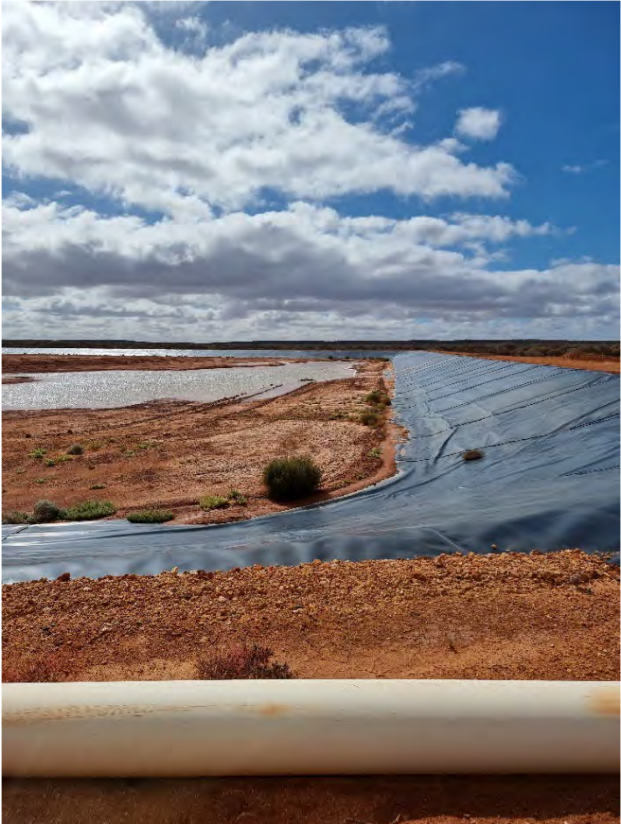
Photo 14. South end of WMP 8 looking North-East
